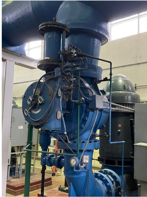
Figure 1: High Service Pump #2 with the existing Allis-Chalmers valve to be removed.
