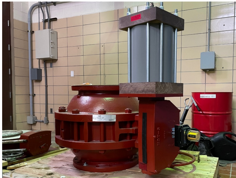
Figure 2: The Henry Pratt 18" rubber-seated ball valve procured by the City for installation on High Service Pump #2.
