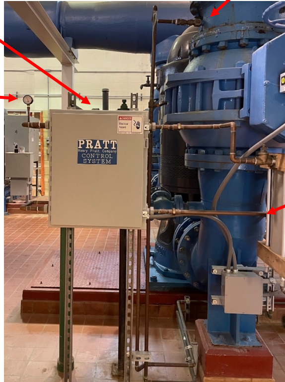
Figure 3: Existing Pratt control system on High Service Pump #1, similar to what will be installed on High Service Pump #2.
